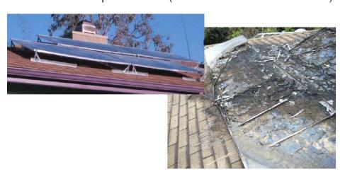
Flat roof with false static, inappropriate material, inexperienced installer
